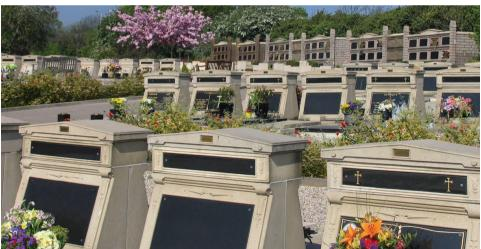
Their development of the mausolea interment unit allows **welters**® to provide both front and side charging options as shown. These units dominate the section and are also utilised as retaining structures, allowing the ground level to change. The ground level behind the mausolea is ~1m higher than that at the front.
