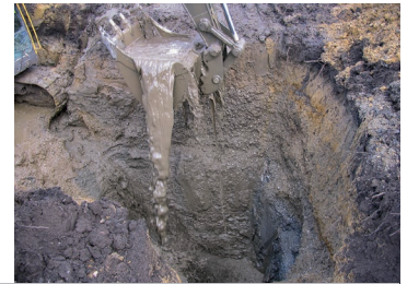
BEFORE - examples of the excavated material and accumulated rubbish found on sites being developed by welters, unsuitable for earthen burial
