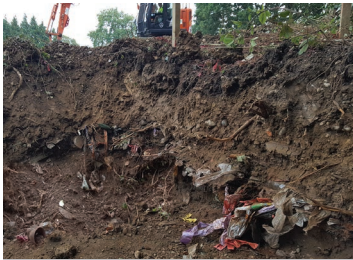
BEFORE - examples of the excavated material and accumulated rubbish found on sites being developed by welters, unsuitable for earthen burial
