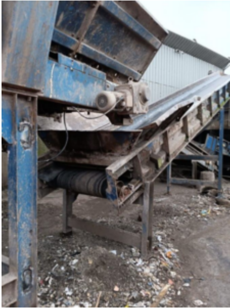
The unguarded conveyor
