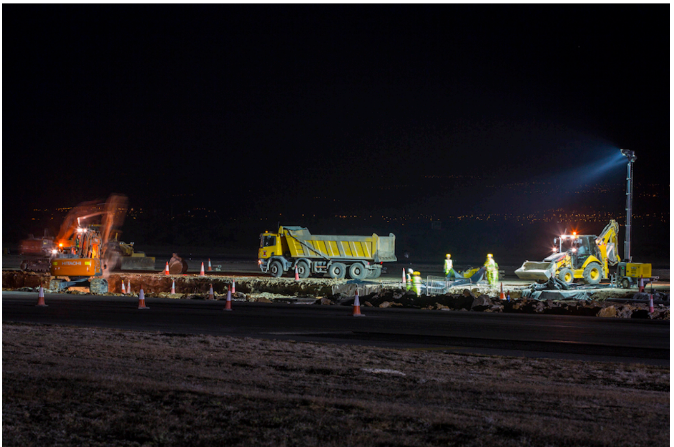
Night time work on the RAF Akrotiri runway.
