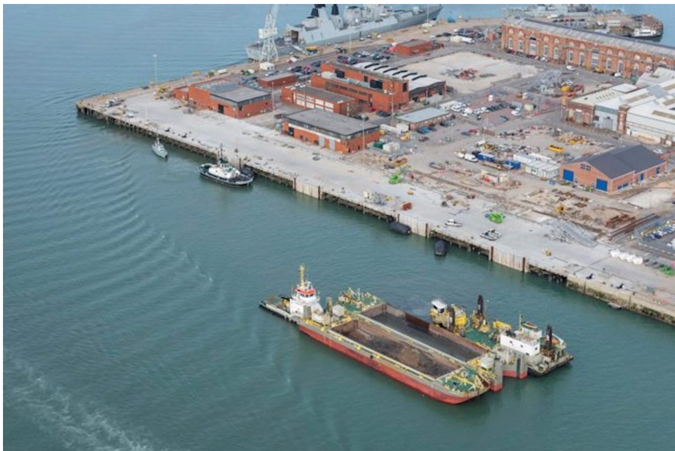
The Princess Royal Jetty from above
