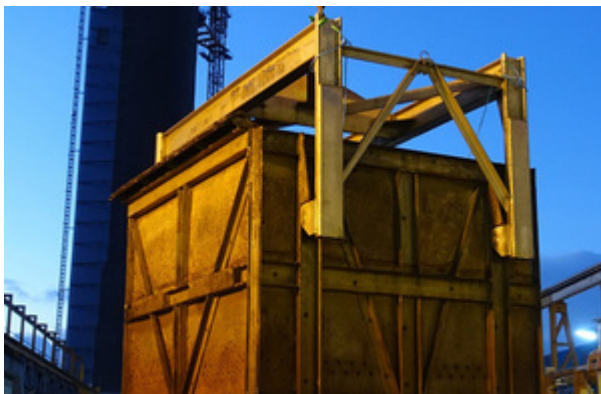
Skip being retrieved from the Pile Fuel Storage Pond at Sellafield
