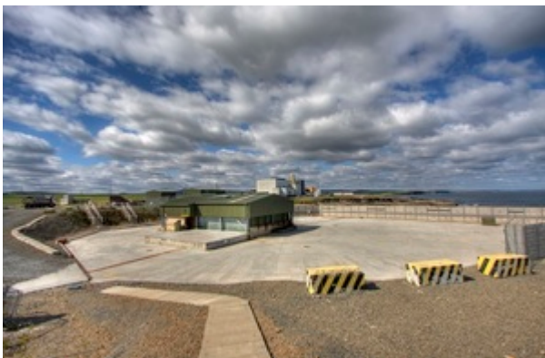
The Dounreay shaft
