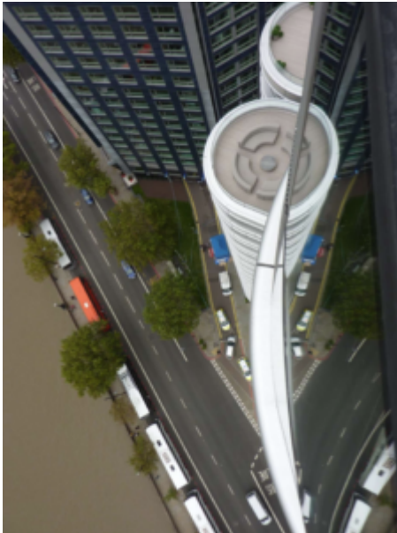
Another taken by HSE showing height of penthouse
