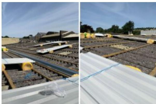
The man fell through a fragile rooflight while carrying out over-cladding work
