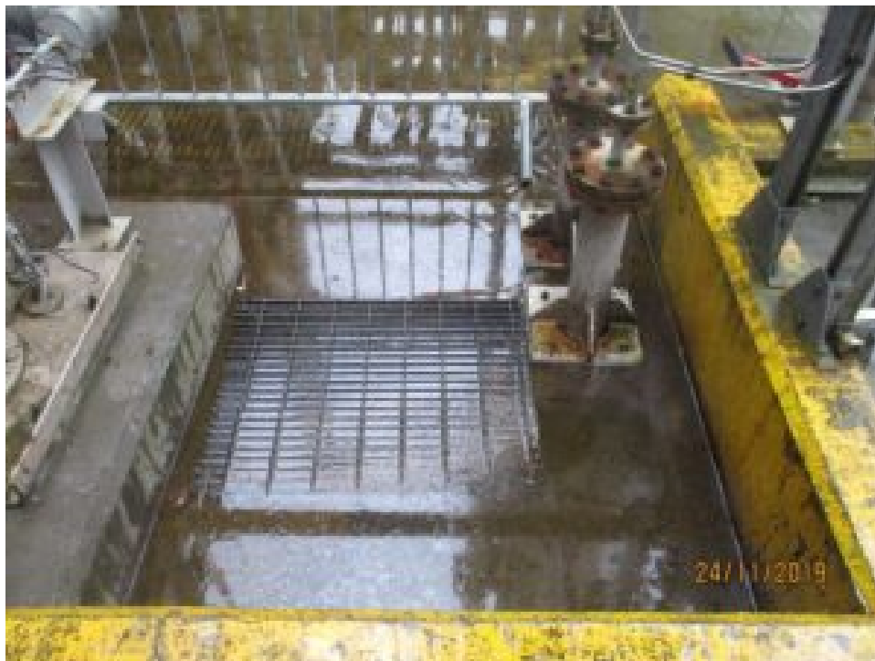
Photo of sump with grating in place taken shortly after the incident
