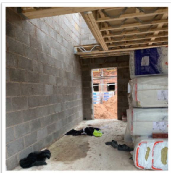
The open stairwell
