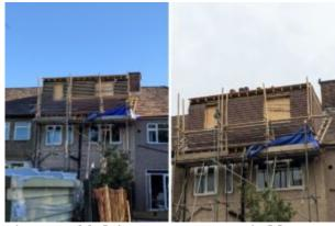
The scaffold was a potentially dangerous structure at risk of collapse and in breach of the HSE prohibition notice.
