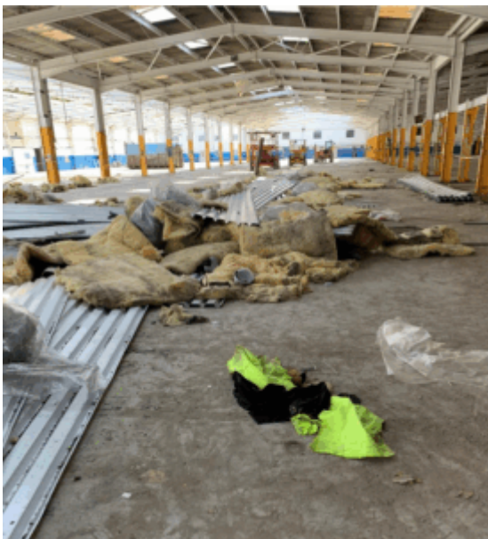
Warehouse in question
