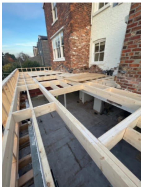
Work area where the incident occurred
