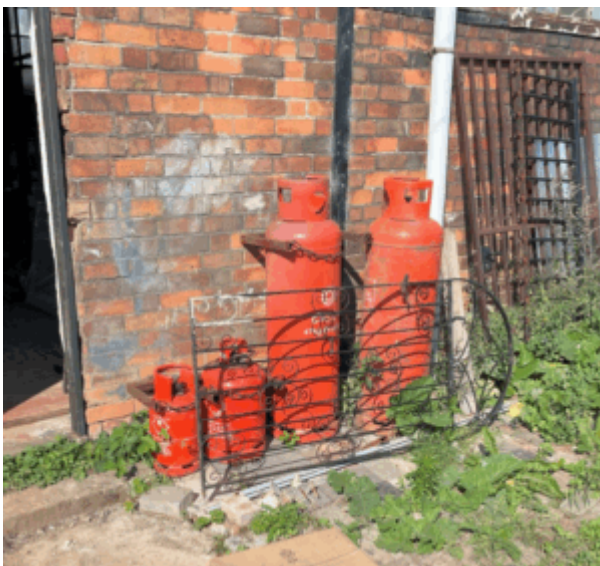
Unsafe storage of flammable gas
