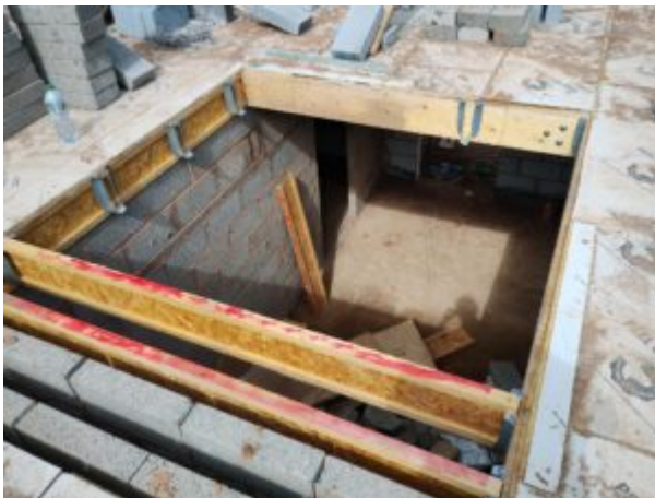
The collapsed stairwell after the incident
