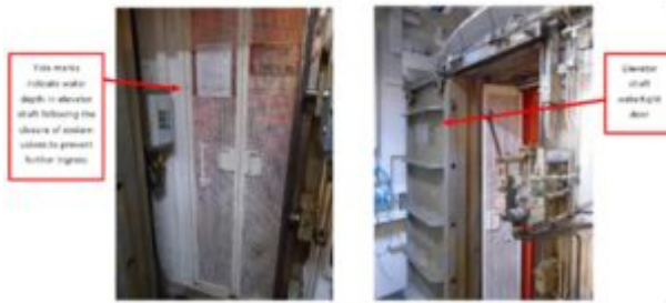
Figure 11 – Lift Entrance and Waterlight Door in P-M-12
