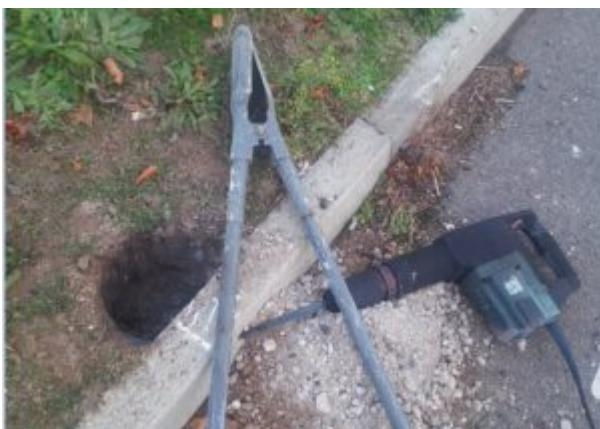
While operating the electric breaker, one of the operatives struck an 11kv electricity cable causing a large flash and engulfing him in flames. The operative sustained serious burns to his face, chest, abdomen, groin, both arms and both legs, amounting to approximately 50% total body surface area burns.
