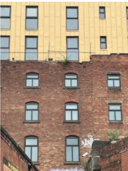
Rear of 35 Glovers Court Preston showing exposed RSJs, cracks and missing coping
