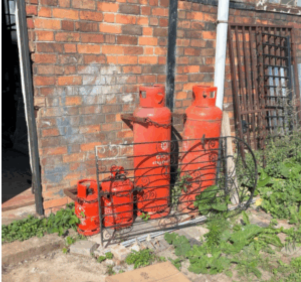
Unsafe storage of flammable gas
