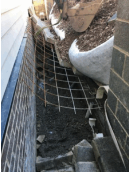
Collapsed wall
