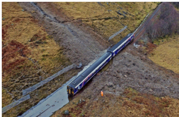
Aerial image of the landslip and derailed train
