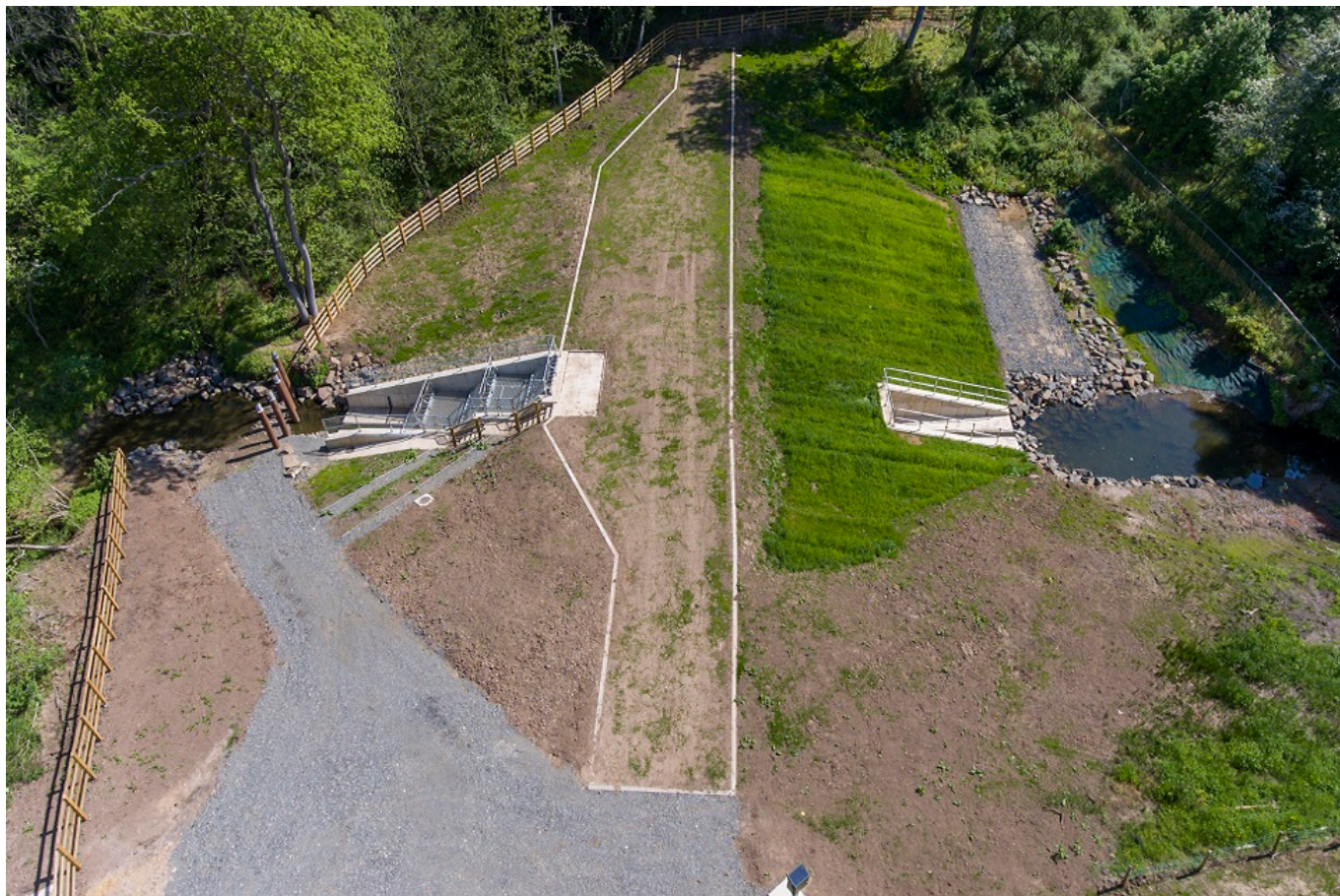
Cotting Burn dam aerial image
