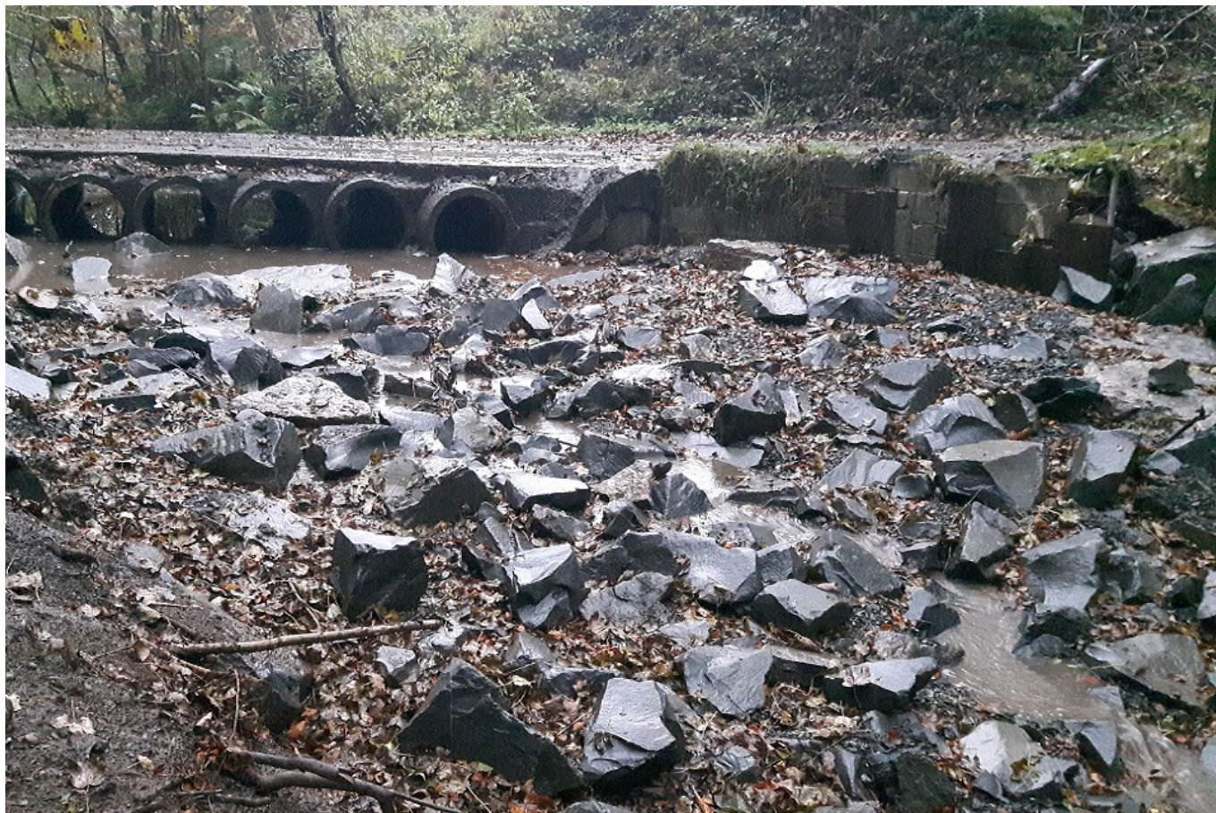
The newly constructed rock ramp at Brancepeth Beck
