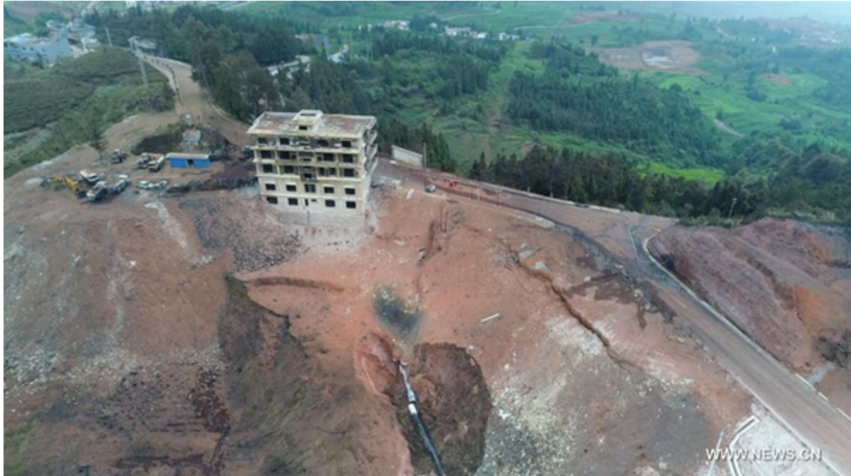
The site of a gas pipeline explosion is seen in Qinglong, southwest China's Guizhou Province, July 2, 2017. [Photo/Xinhua]
