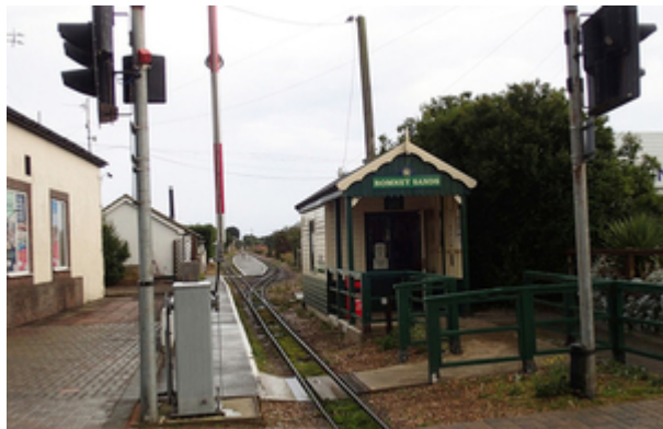
Romney Sands ticket office and station platform
