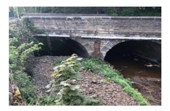
Gravel deposits have built up at the bridge and will be removed as part of the work.
