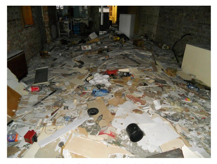
An investigation by the Health and Safety Executive (HSE) found that a management asbestos survey and a refurbishment and demolition asbestos survey had not been completed prior to the work starting, and the work had not been completed by a licenced asbestos contractor.
