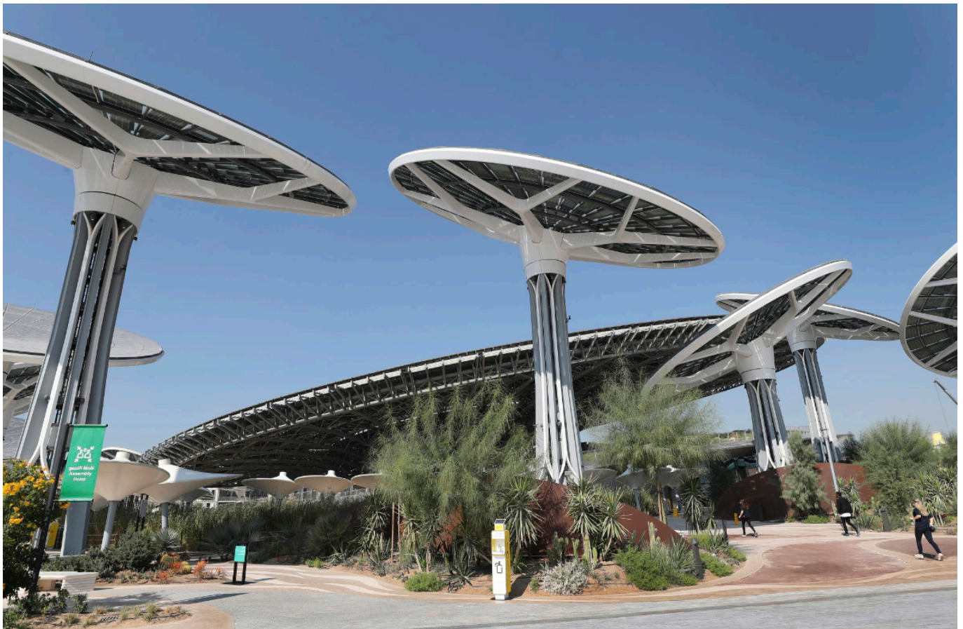
A view of Terra, The Sustainability Pavilion at the Dubai World Expo site in Dubai. (AP Photo/Kamran Jebreili)
