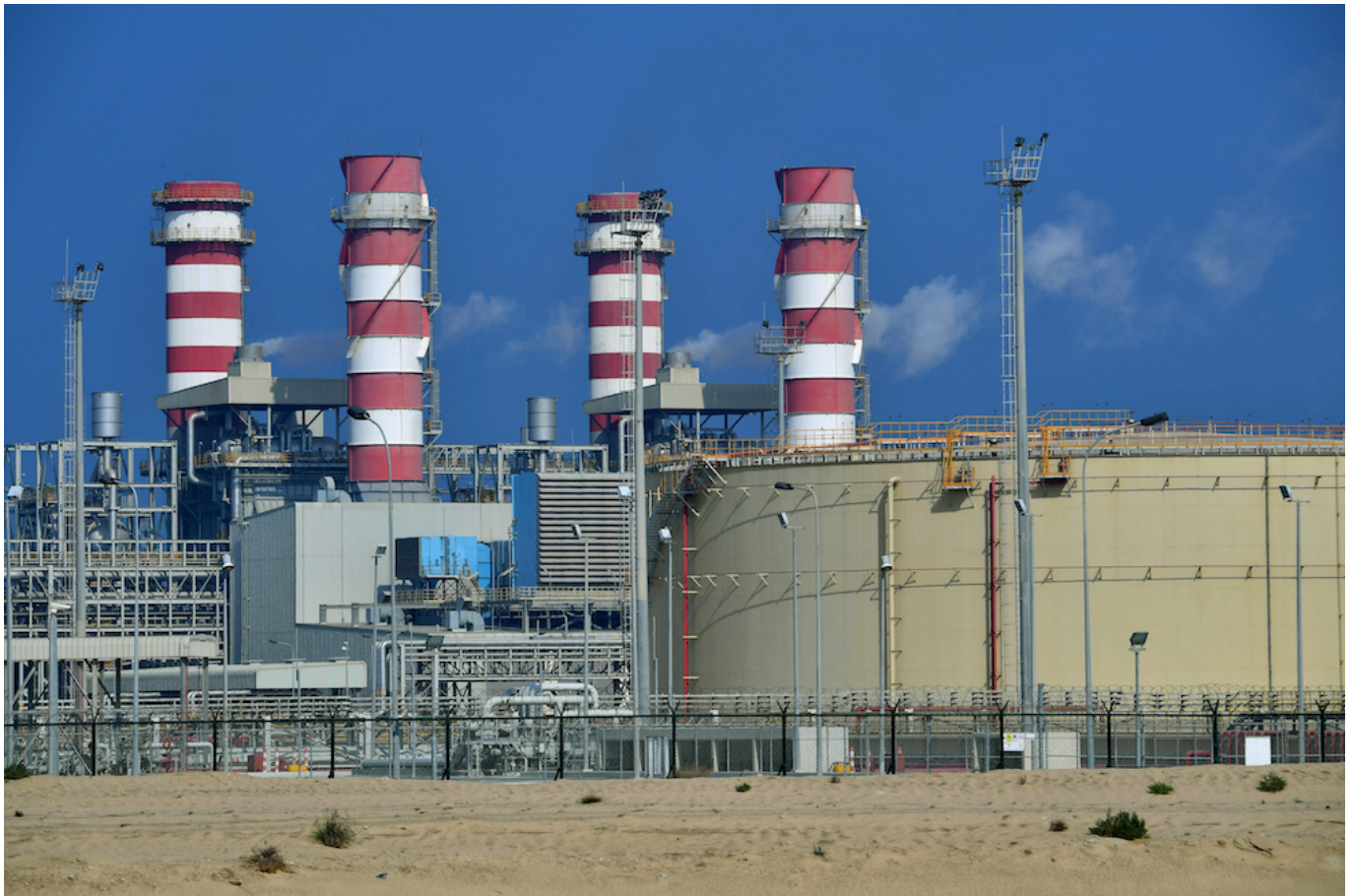
A view of Jubail Desalination Plant at the Jubail Industrial City, about 95 kilometers north of Dammam in Saudi Arabia’s eastern province. (AFP/File Photo)
