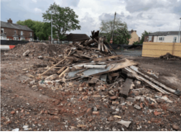
Property demolition site of former pub
