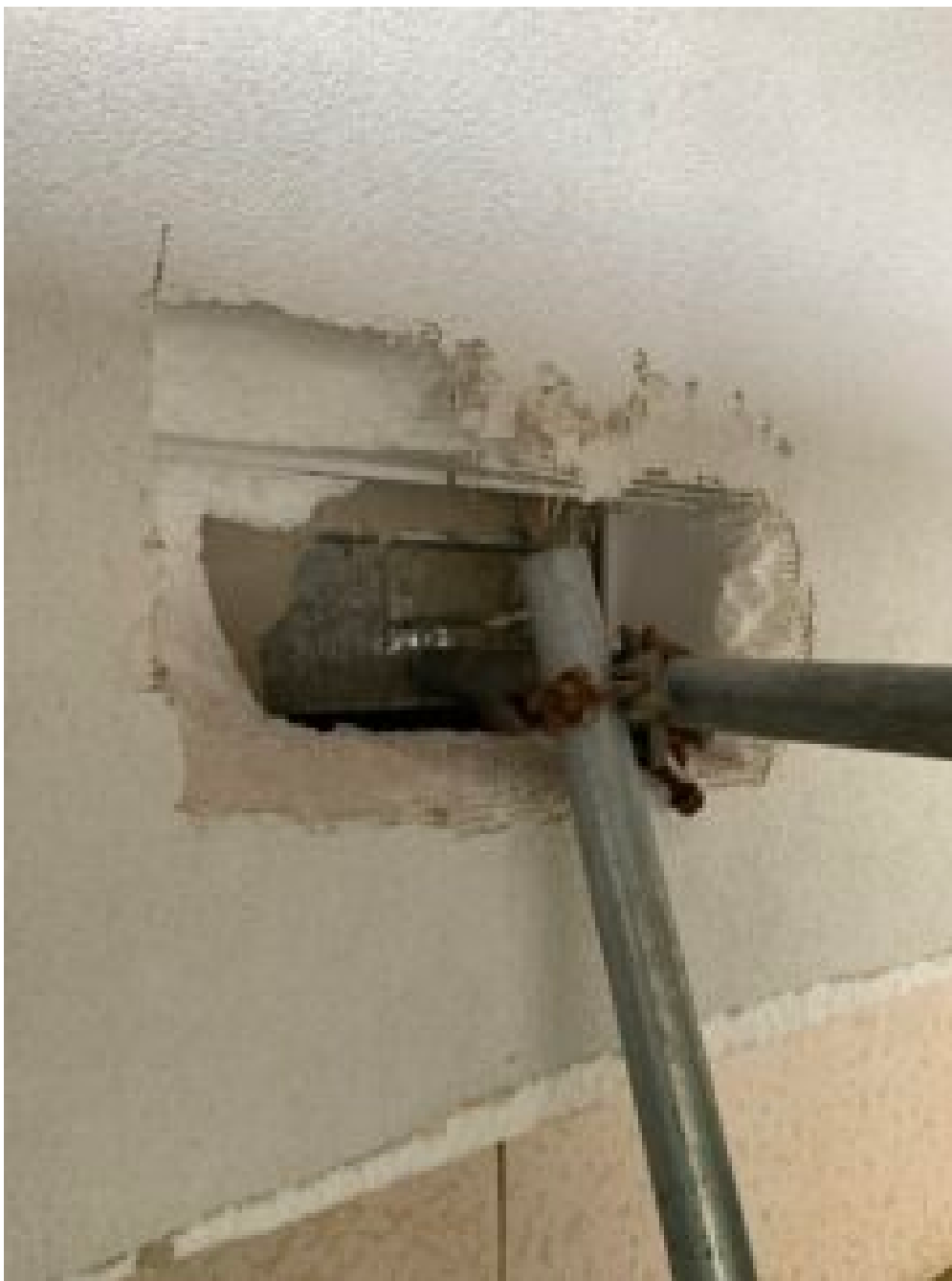
Combustible material exposed where scaffold is attached
