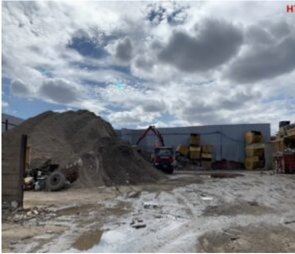
Skips were stacked in an area regularly accessed by workers
