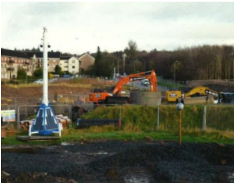
The construction site adjacent to Glenkirk Drive
