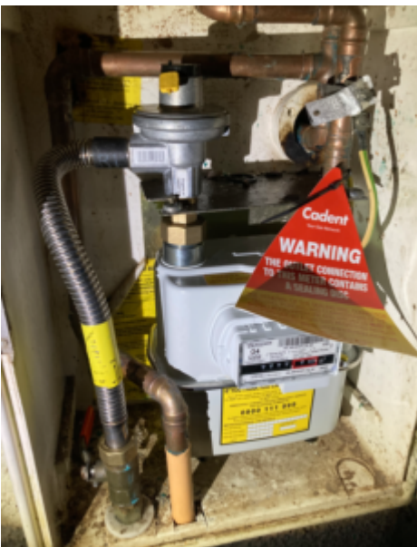
The meter box following the gas supply being capped
