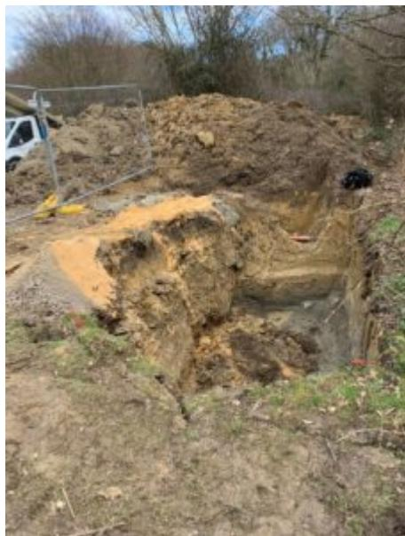
The three men were working in this excavation when it collapsed
