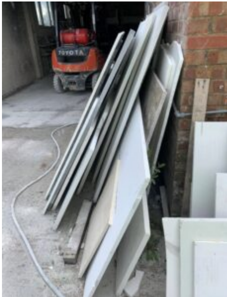
Heavy stone slabs were not being stored safely
