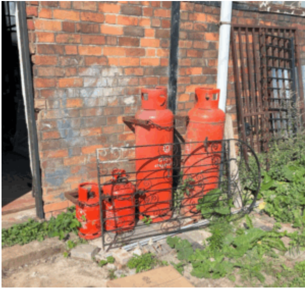
Unsafe storage of flammable gas
