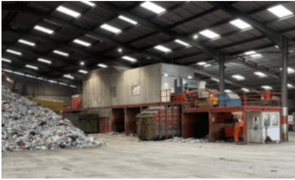
Machinery at the site at Aycliffe Quarry
