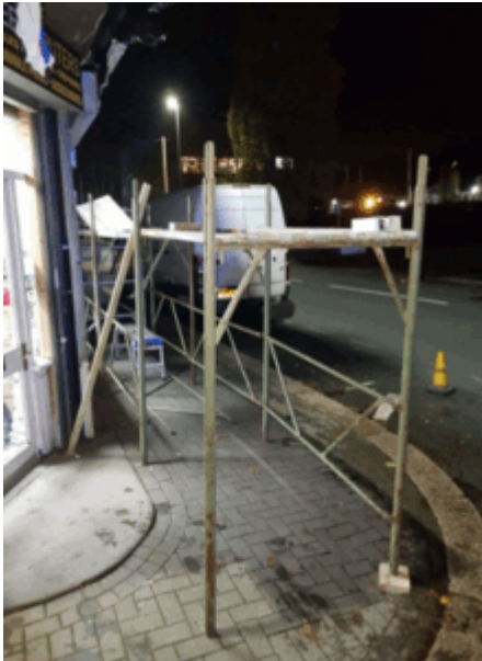
The scaffolding tower without edge protection
