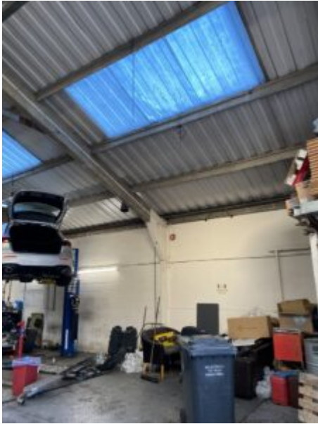
Skylight and area below
