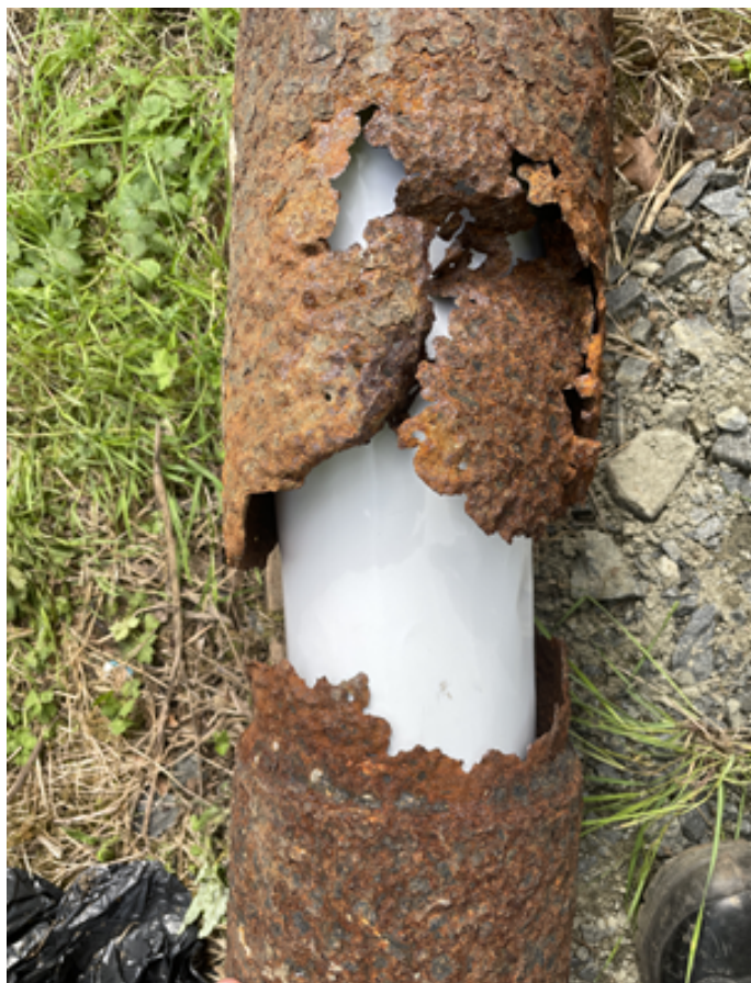
Image of the corroded lamppost following the collapse
