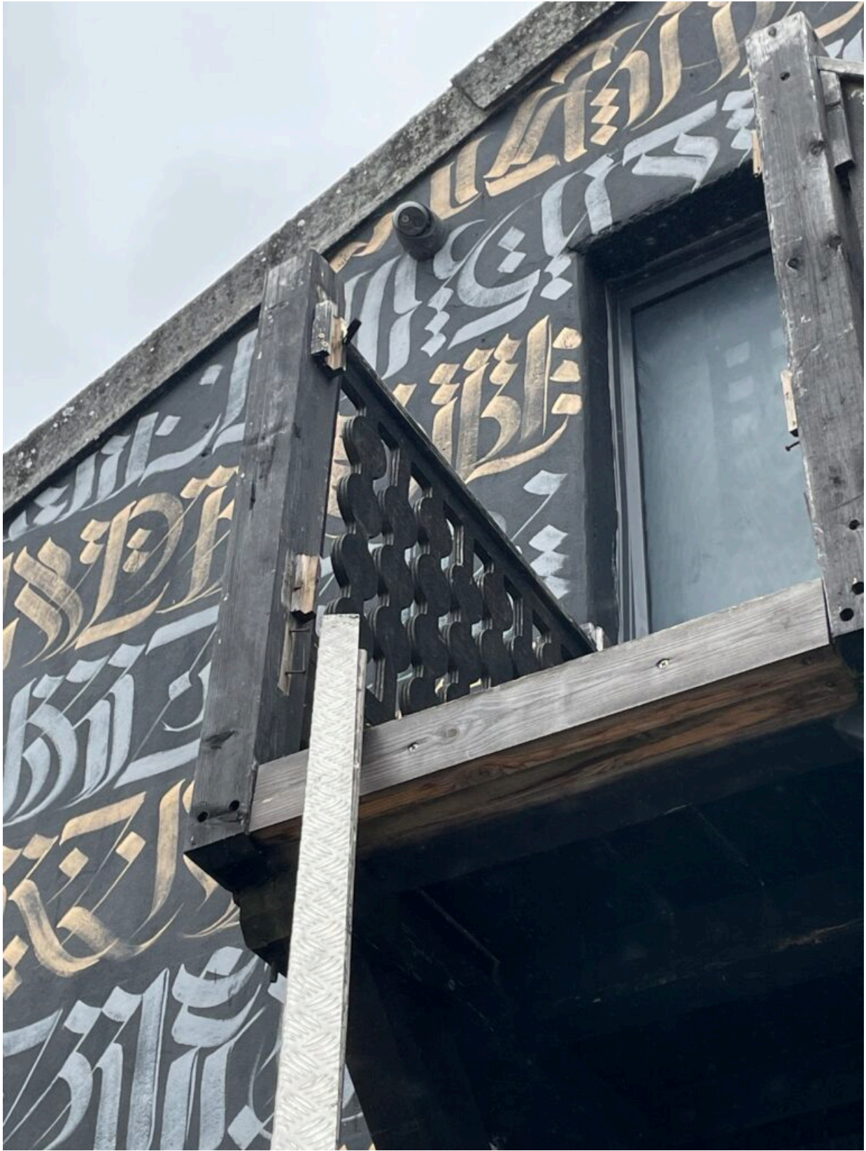
Image of staircase
