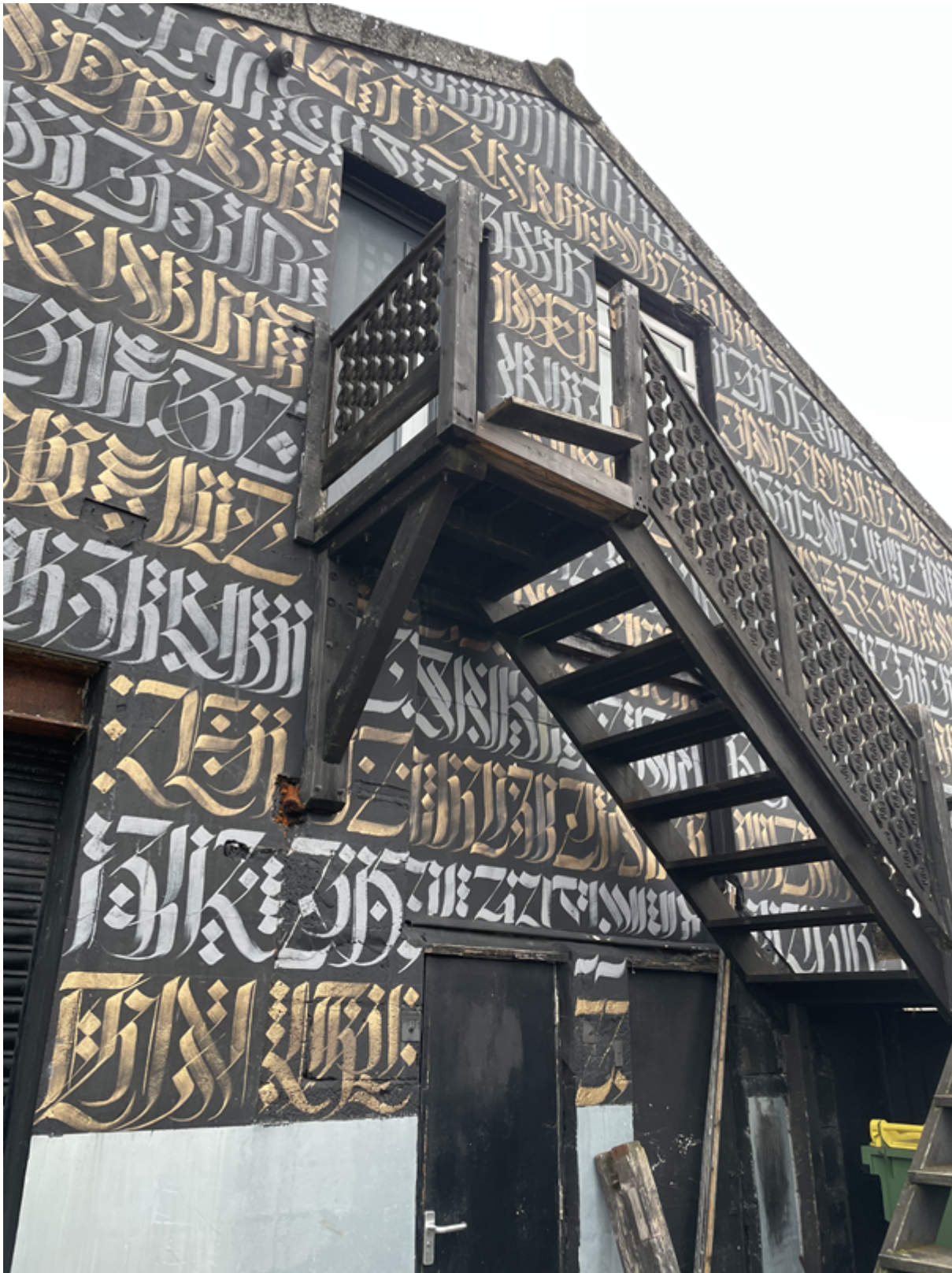
Image of staircase
