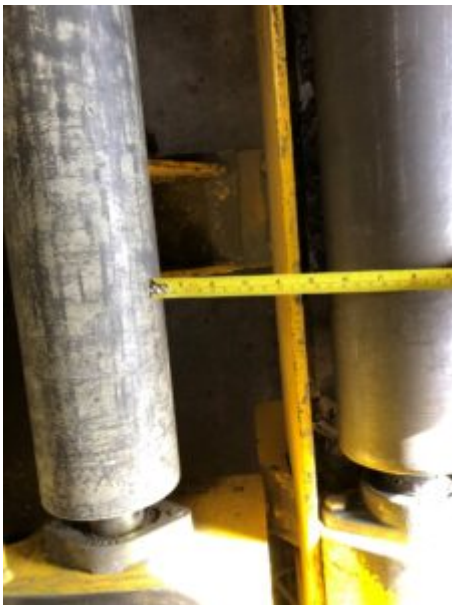
Photo of gap in roller deck pre-accident
