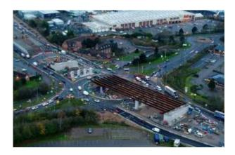
The new steel beams being installed at Binley junction in Coventry
