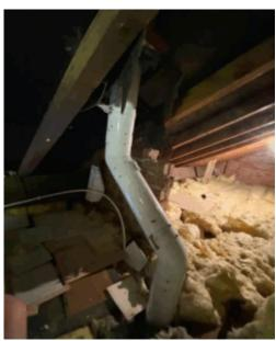
Defects included a lack of support for the chimney and flue system
