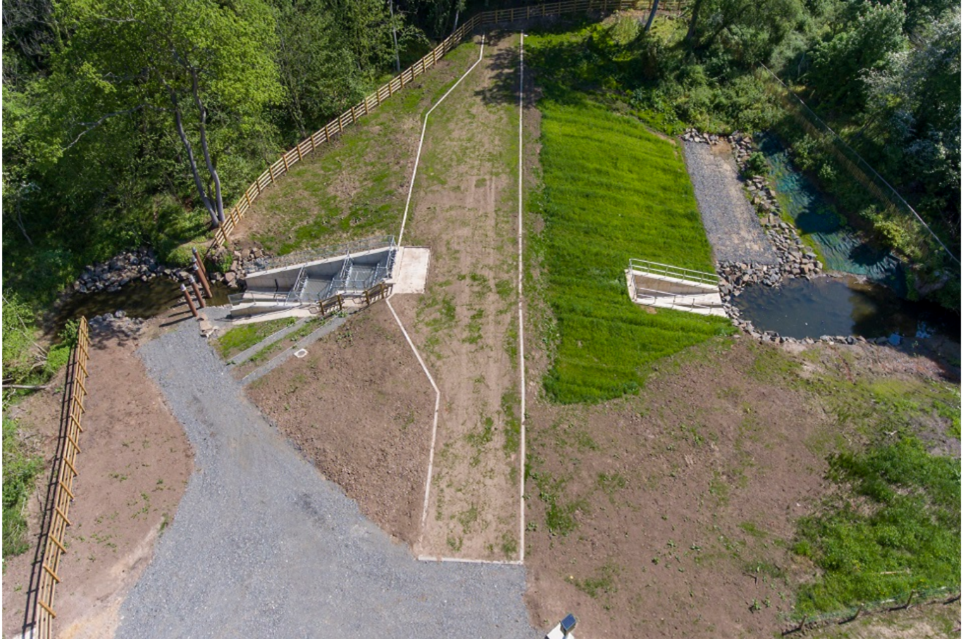
Cotting Burn dam aerial image
