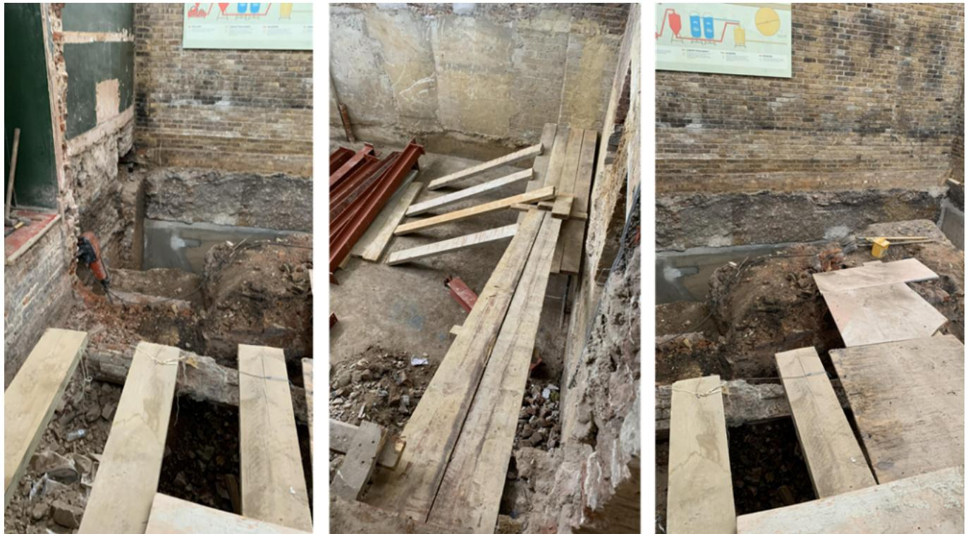
Images from site show poor work at height practices and failures to suitably plan, manage and monitor the construction work.
