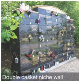
Double casket niche wall
