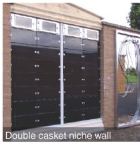
Double casket niche wall
