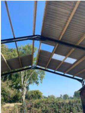
Partially constructed barn in Shropshire worker fell from An investigation by the Health and Safety Executive (HSE) found that Dewi Williams Limited failed to properly plan the work and to put in place measures to prevent or protect against a fall from height.
