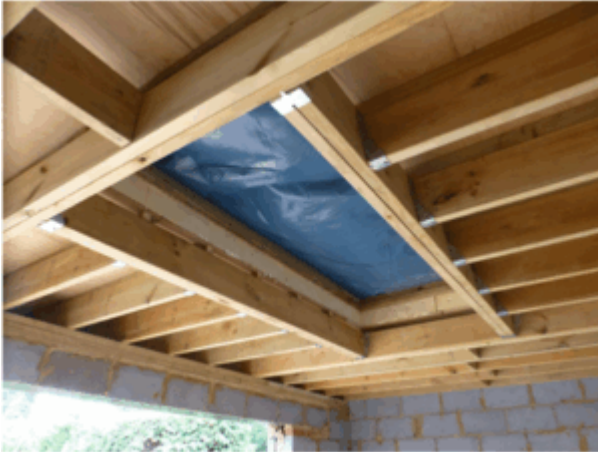
Tarp covering roof/hole when HSE attended
